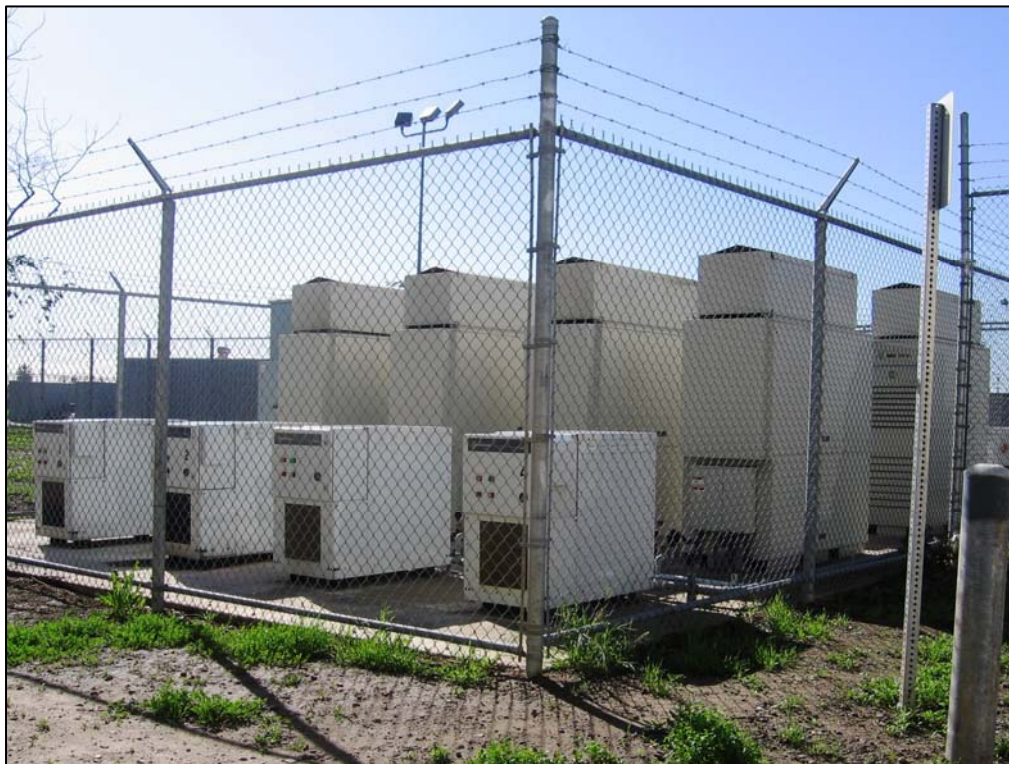
The turbines above are rated at 60KW (thousands of watts) each and provide an actual supplement of between 30KW and 60KW per turbine to the Southern California Edison feed at the Data Center.
